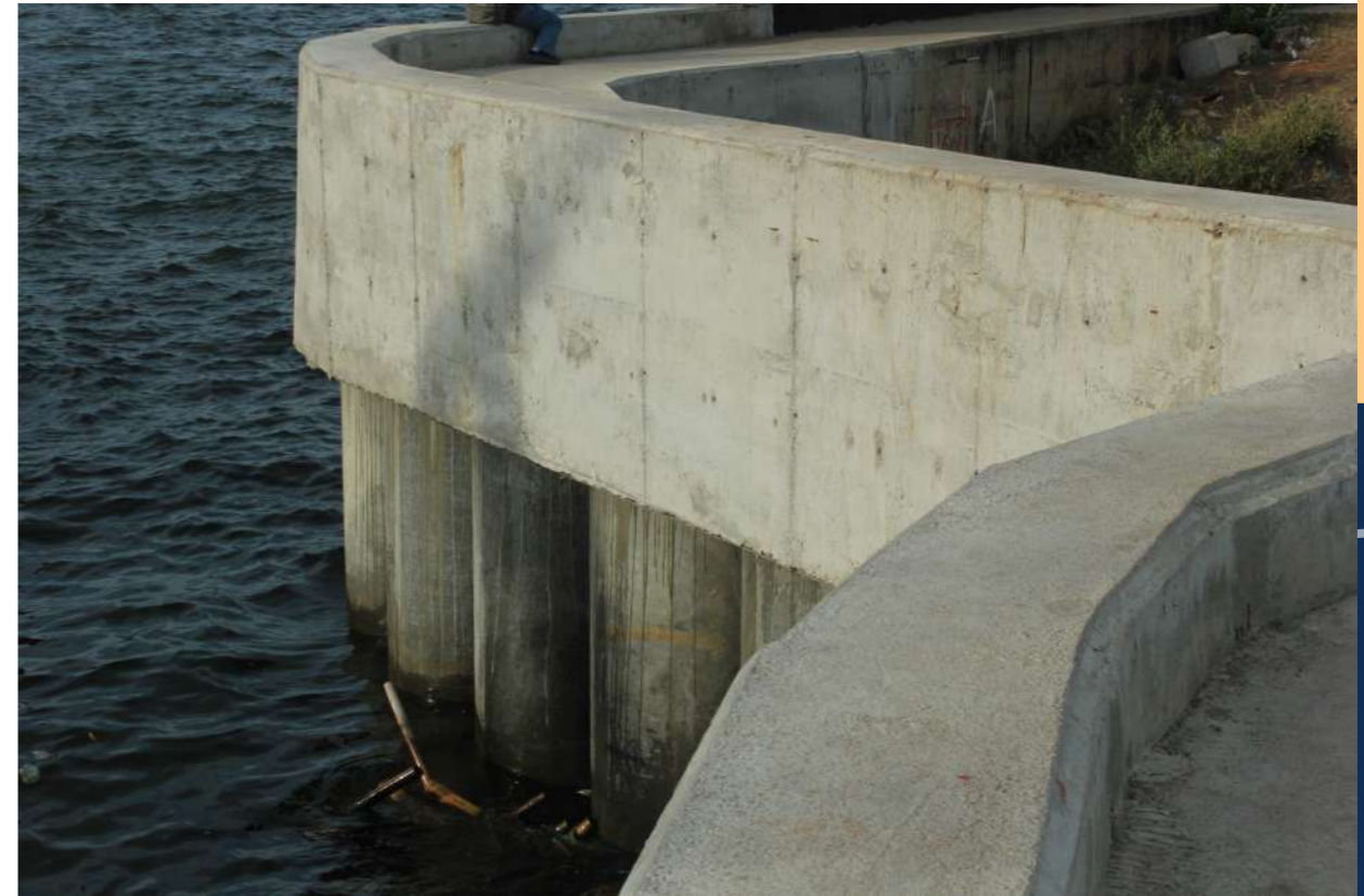
Tanggul Besar, 2022 The Giant Sea Embankment, 2022
